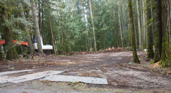
After the logging, clearing and leveling
