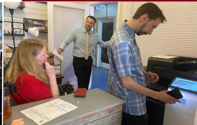
Kasey oversees install of our new Konica copier.
