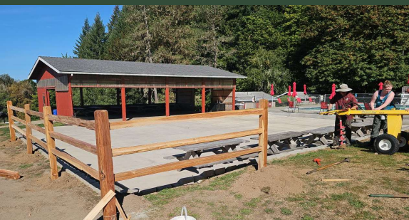
The new Picnic Pavilion fence adds a sense of comfort and safety to the concrete pad.
